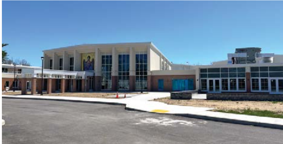
VIEW OF ENTRANCE AND FACADE
