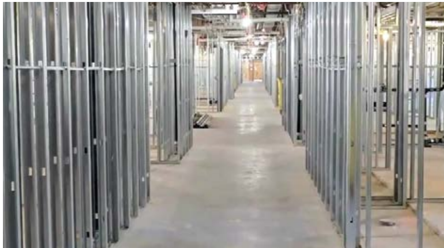
ASSISTED LIVING MAIN CORRIDOR - GROUND FLOOR
